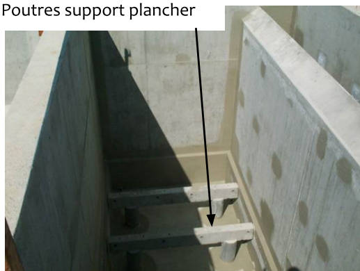
Poutres support plancher
