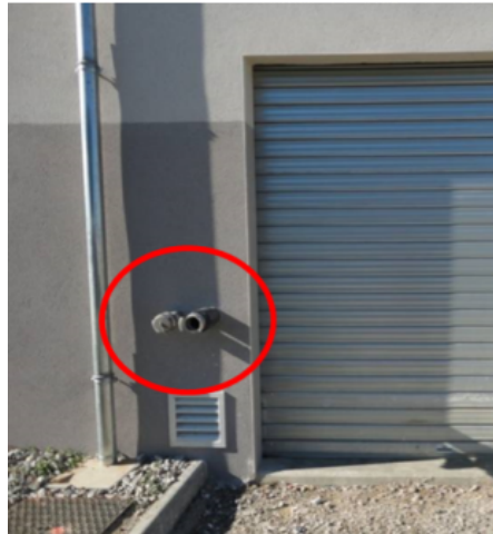
EXEMPLE RACCORD COTE RACCORDEMENT CAMION
