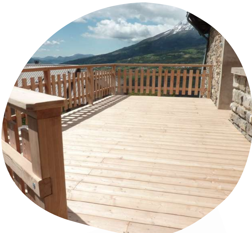
Terrasse bois – Source: eco 2 SCOP
