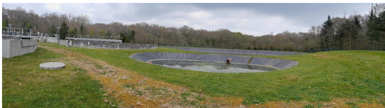
Figure 1. Station d'épuration de Combrit (Source : ©Biotope)
