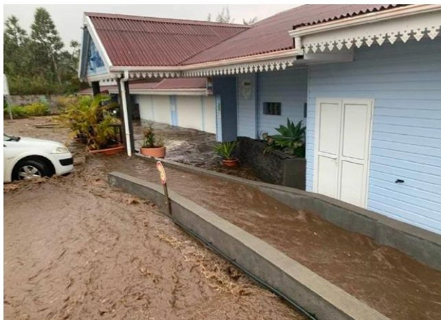
Inondation, Saint-Philippe – RN2 (2021)
