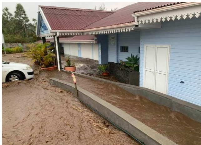
Inondation, Saint-Philippe – RN2 (2021)
