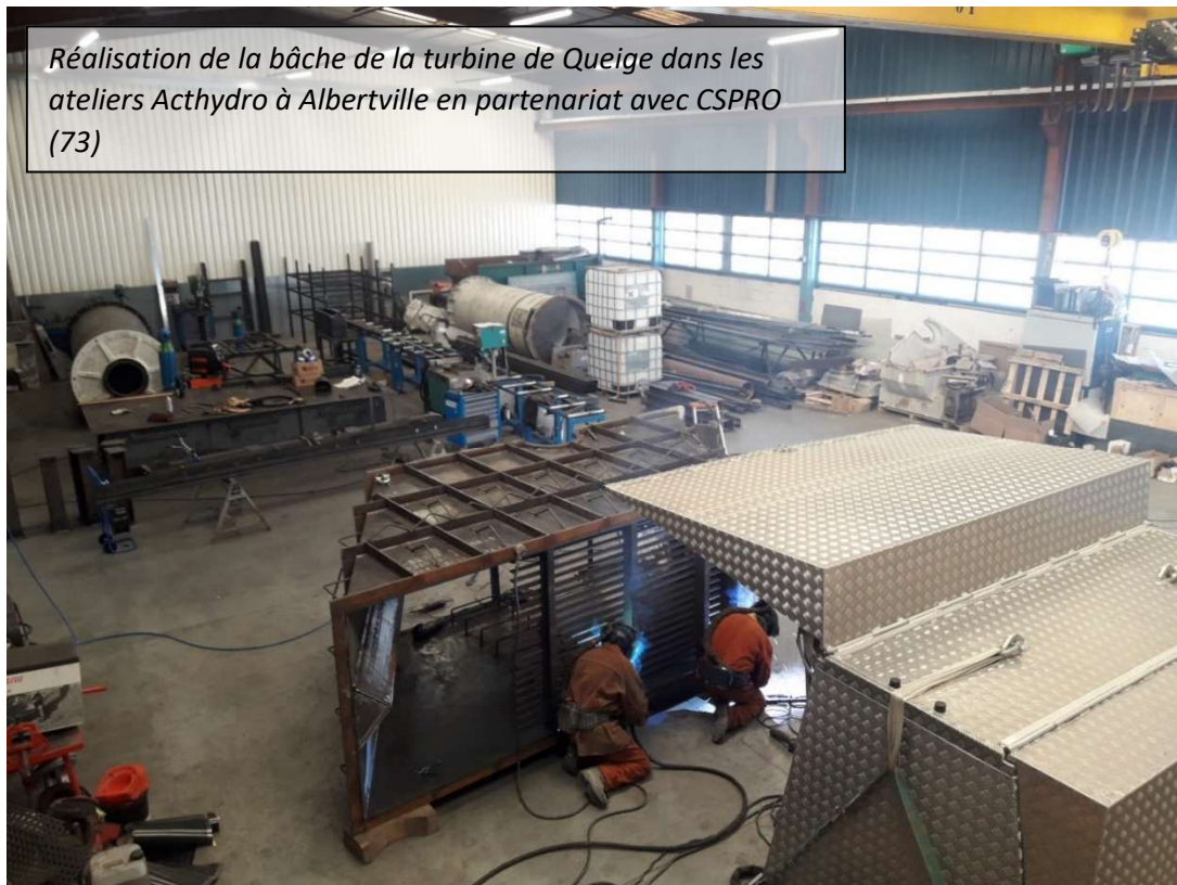
Figure 2: atelier de construction
