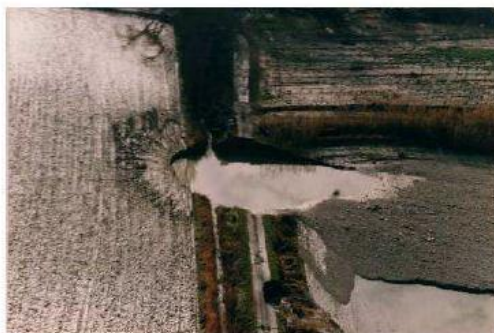
Figure 129 : Rupture de l'épi du village (Puget, 13)
