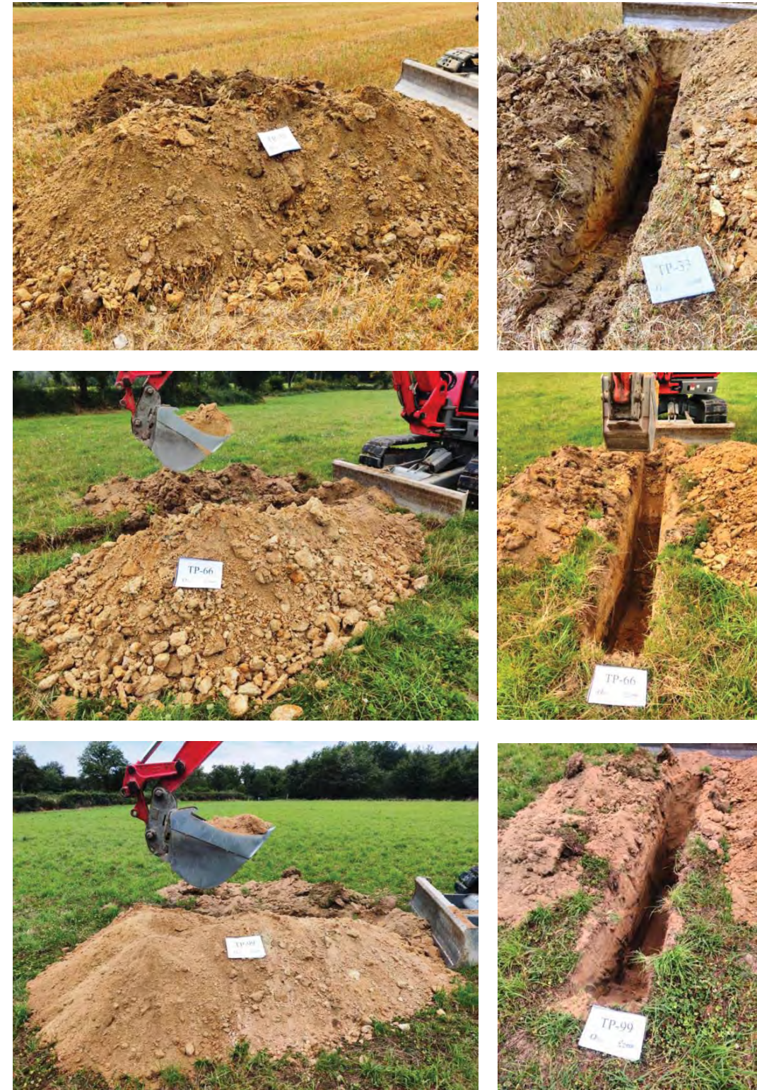
Photo 1: Soils excavated in some of the trial pits
