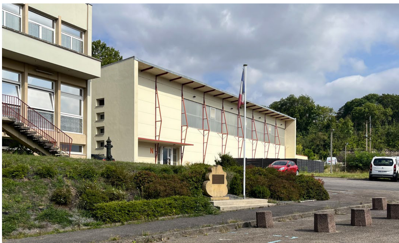
Figure 48: Photos de site ATELIERS 2/3/4/ - OTE - OTELIO - EXPUR, 2025
