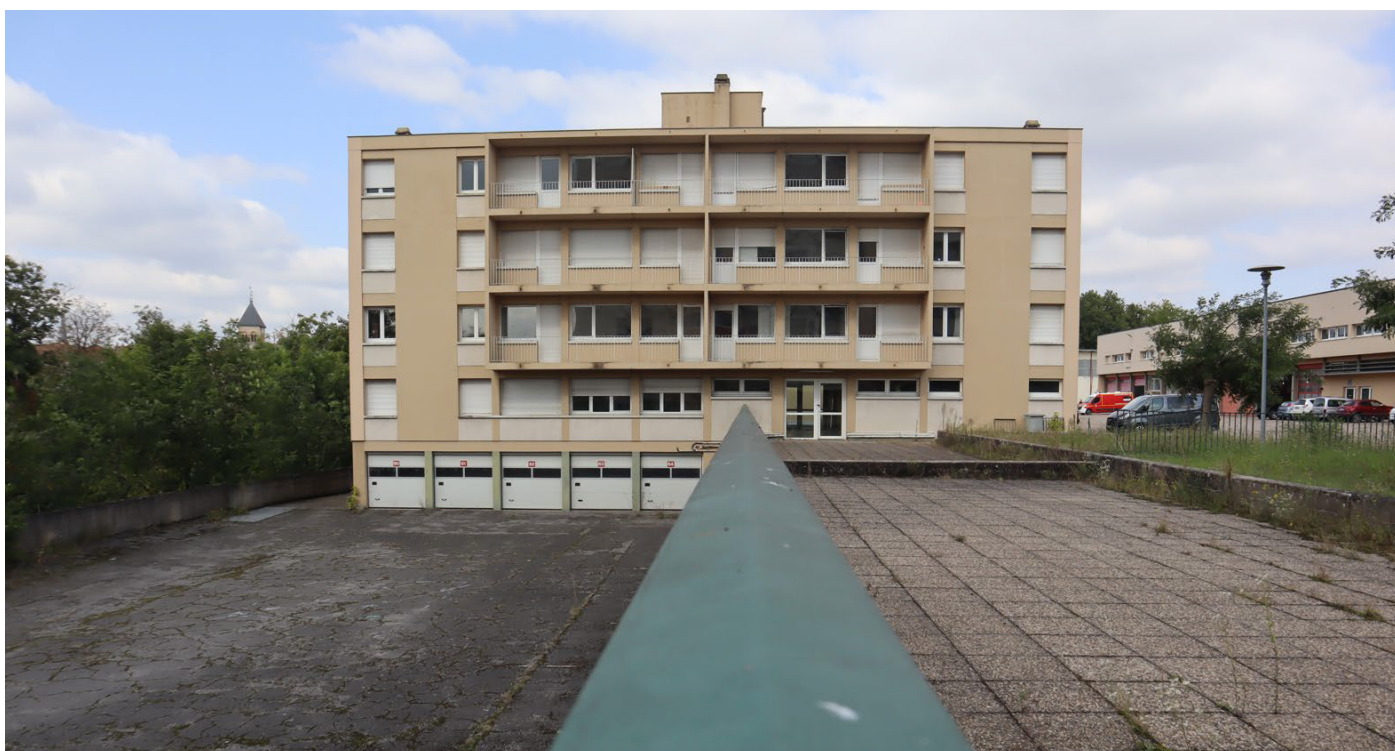
Figure 46: Photo de site ATELIERS 2/3/4/ - OTE - OTELIO - EXPUR, 2025
