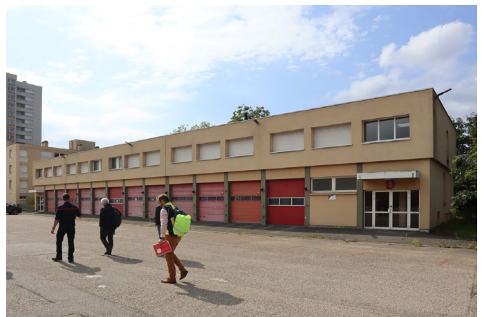
Figure 43: Photos de site ATELIERS 2/3/4/ - OTE - OTELIO - EXPUR, 2025
