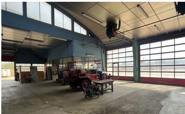
Figure 44: Photos de site ATELIERS 2/3/4/ - OTE - OTELIO - EXPUR, 2025
