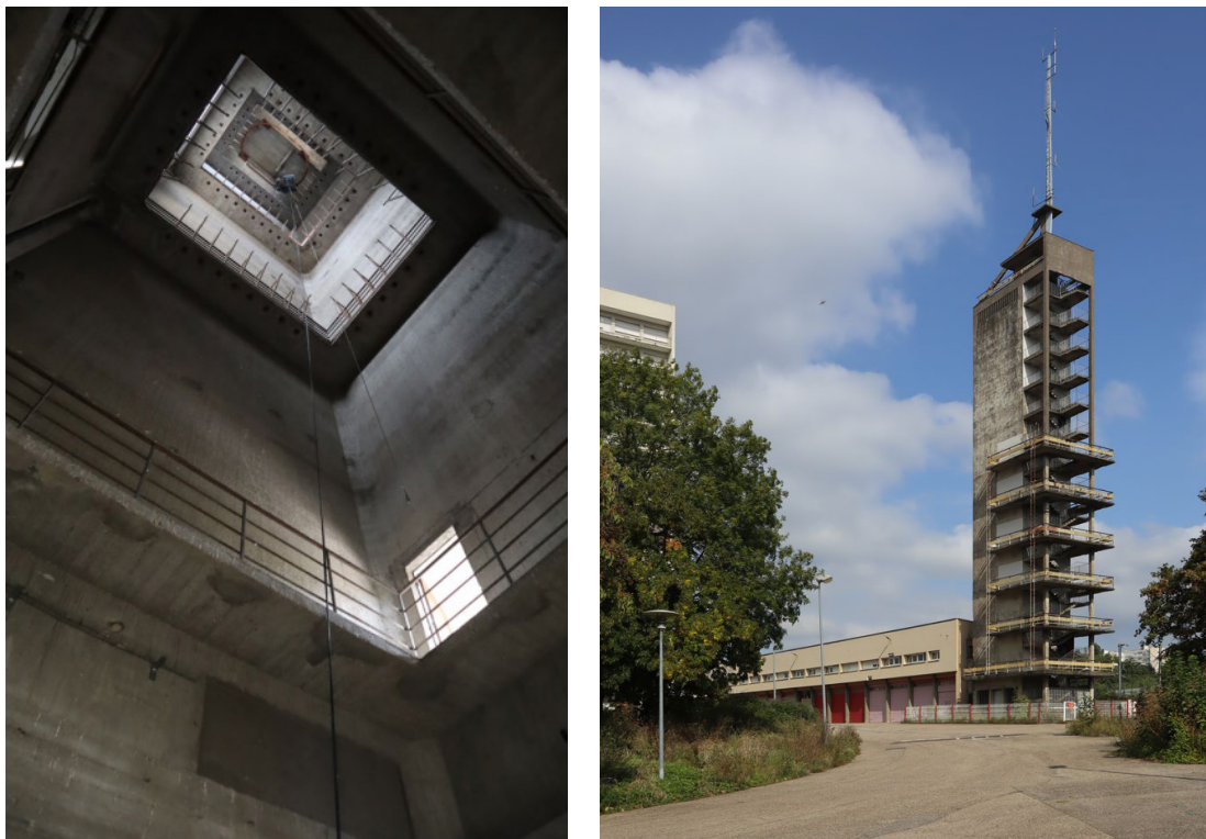
Figure 42: Photos de site ATELIERS 2/3/4/ - OTE - OTELIO - EXPUR, 2025
