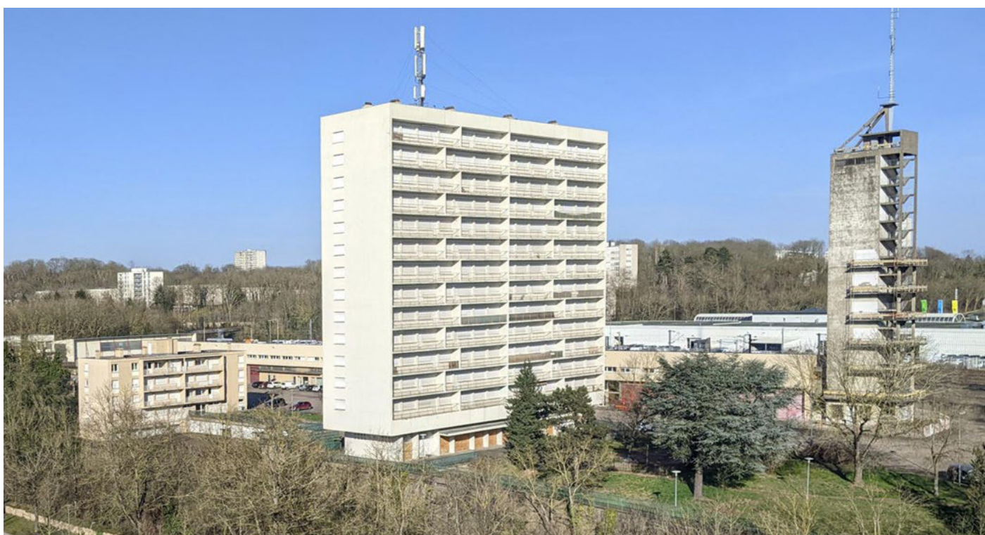
Figure 45: Photo de site ATELIERS 2/3/4/ - OTE - OTELIO - EXPUR, 2025
