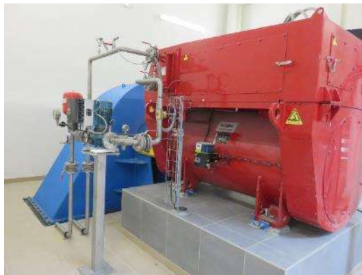
Figure 61..alternateur synchrone
