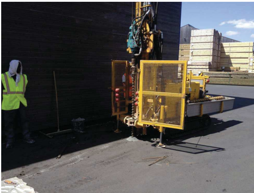
Photo 8. BH7 location at the East of the building
