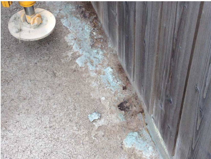
Photo 2. Green coloration on the ground near the BH1 borehole
