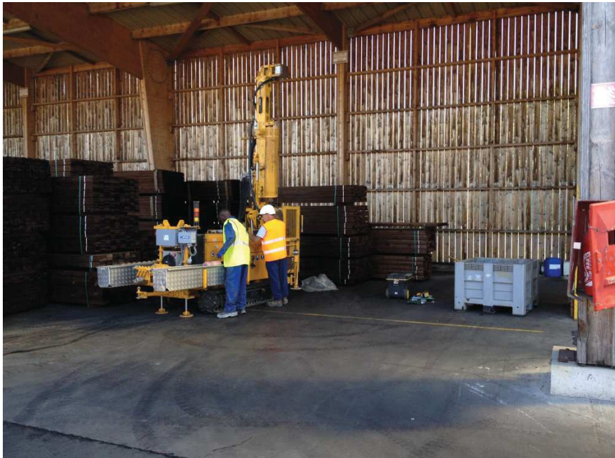
Photo 3. BH2 location at the impregnated wood storage area
