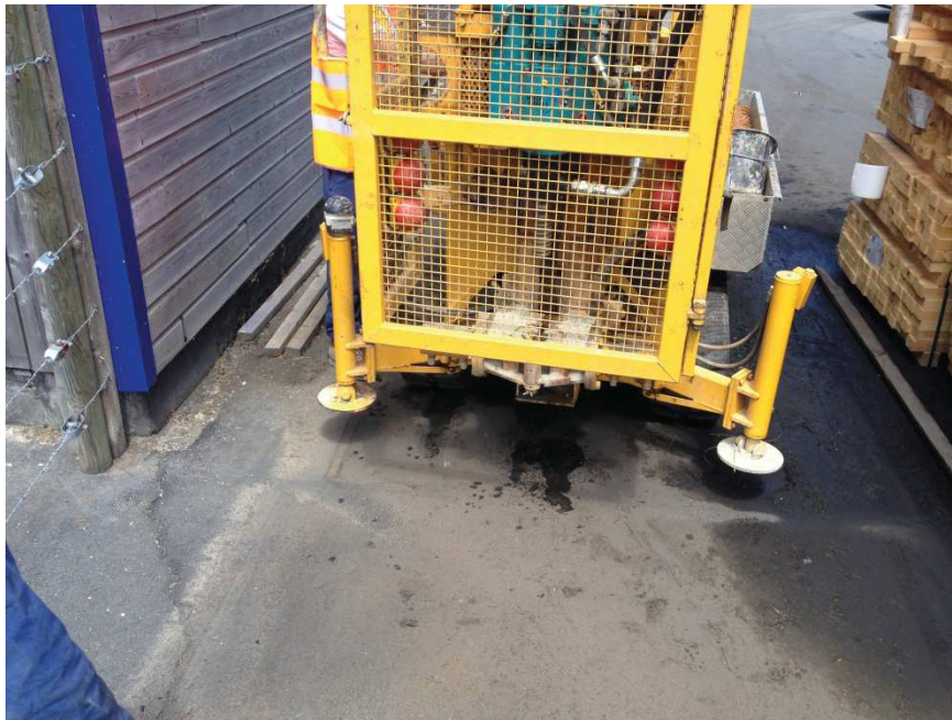
Photo 9. BH8 location at the East angle of the building near an underground collecting tank of the wood impregnating product
