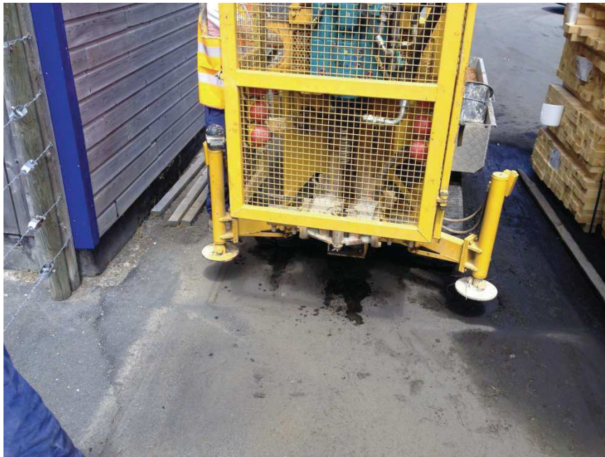
Photo 9. BH8 location at the East angle of the building near an underground collecting tank of the wood impregnating product
