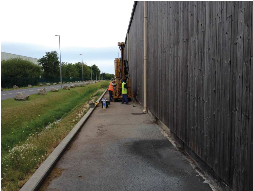
Photo 1. BH1 location at the back of the autoclave building
