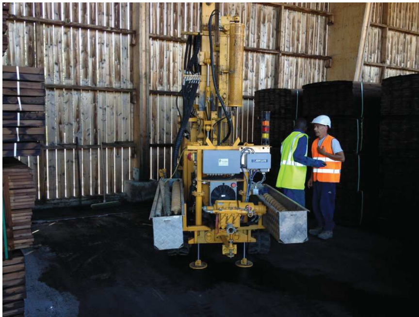
Photo 6. BH5 location at the impregnated wood storage area
