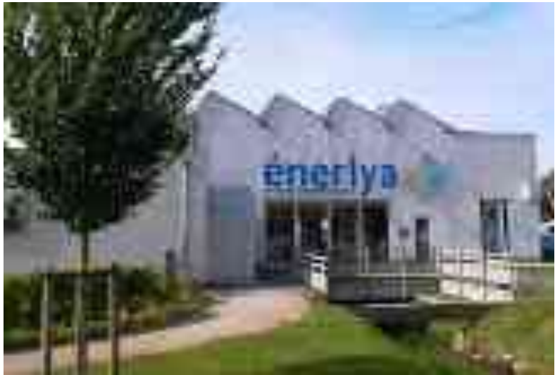
Photo 31 Enerlya (Source : @Enerlya)
