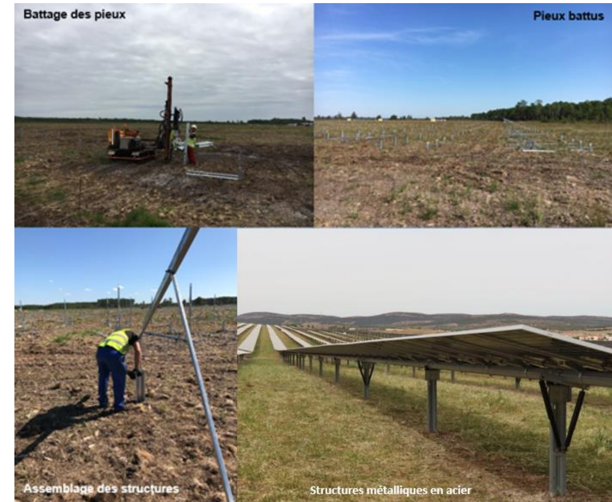
Figure 18 : Structures porteuses - monopieux battus
