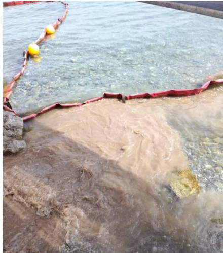
Figure 27 : Illustration des filtres flottant anti-MES
