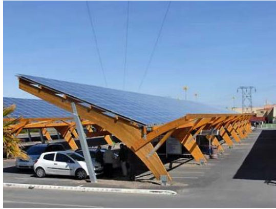
Figure 24: Ombrière photovoltaïque
