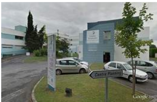
Centre hospitalier (source : Google earth)
