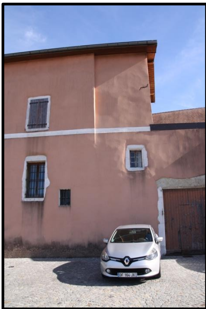
FAÇADE PLACE CDT PERCEVAL
