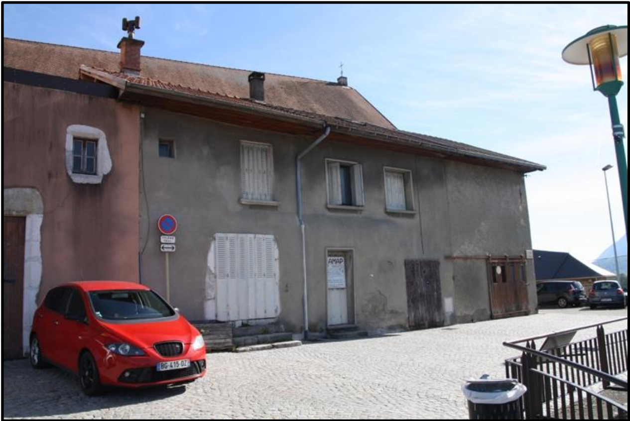
FAÇADE PLACE CDT PERCEVAL
