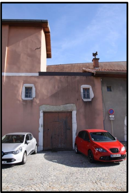
FAÇADE PLACE CDT PERCEVAL
