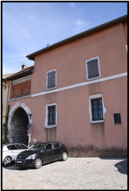
FAÇADE PLACE CDT PERCEVAL
